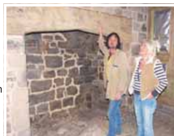
Sue viewing progress with Ian Steele of Shire Oak Construction
