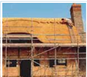
Completing the thatching
