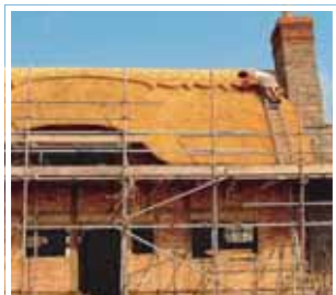
Completing the thatching
