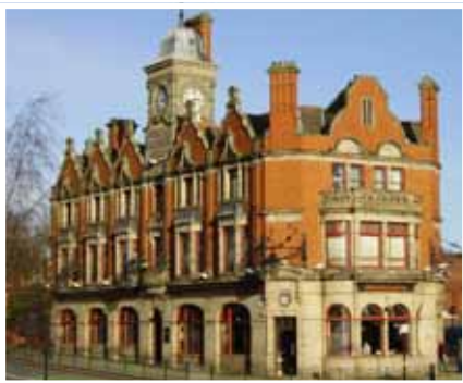
The impressive façade of the Bartons Arms
